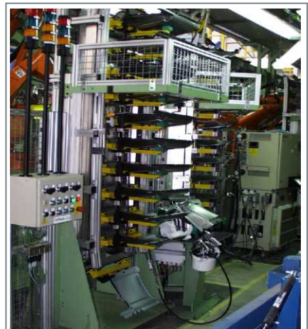
Vertical indexing conveyor Sheet metal infeed for welding cell
